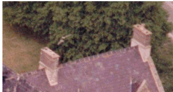
1983 photograph taken before corbels were removed and concrete render applied.
